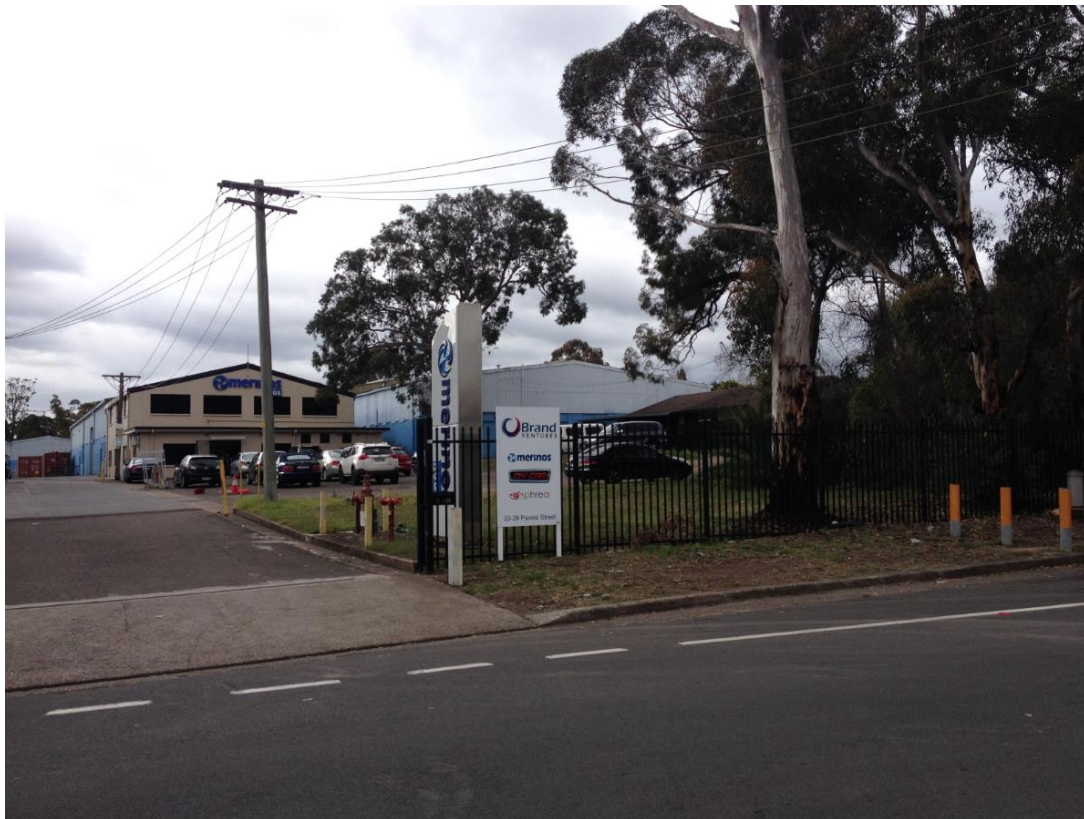
Photograph 2 | 33-35 Pavesi Street from Pavesi Street
