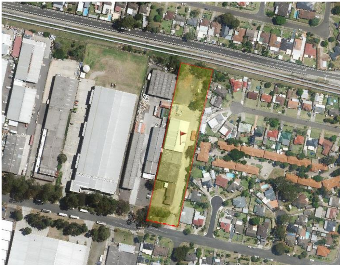
Figure 1| Aerial Site View
