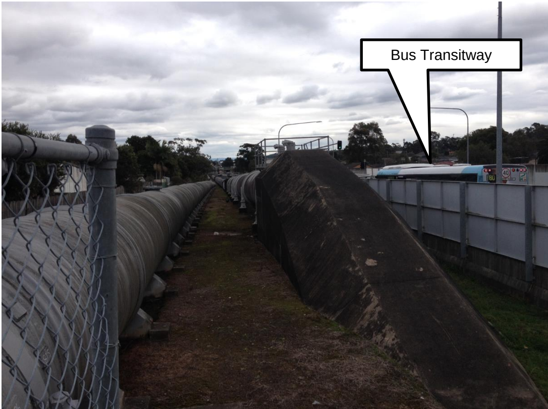
Photograph 6 | Sydney Water pipeline and Liverpool to Parramatta Bus Transitway to north of the Site
