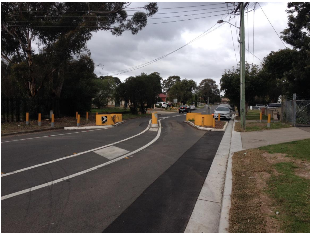
Photograph 8 | Traffic chicane on Pavesi Street (looking east)
